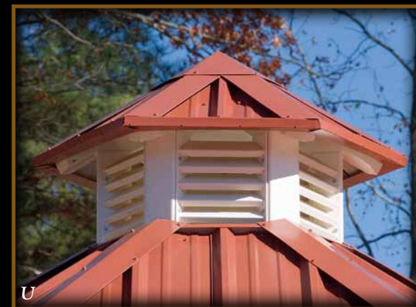
Functional cupola promotes airflow. Shown with R-panel roof. Cupola part of main frame.
