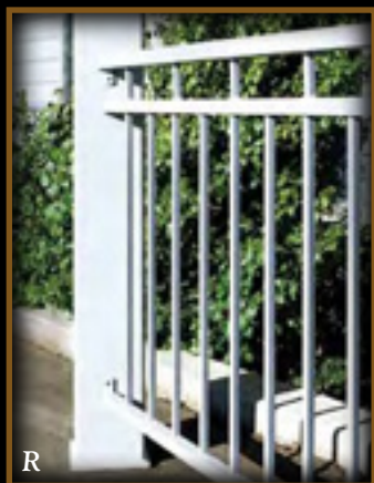
Standard railing with primer paint. Has 5/8" square pickets spaced 5" o.c.
