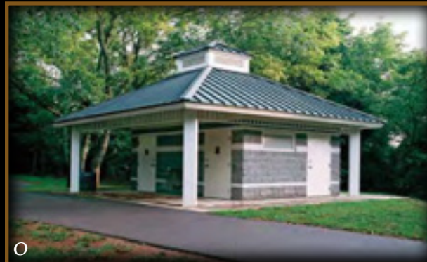
O Knoxville, TN: 22' 6" x 22' 6" custom covers a site-built block restroom. Cool Weathered Copper standing seam roof.
